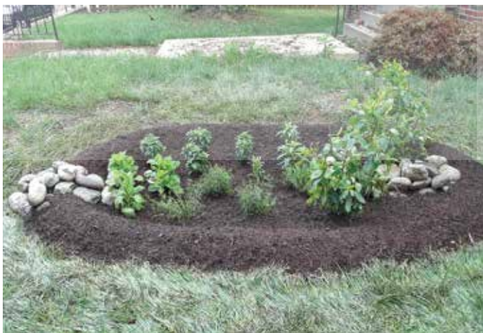
A newly installed RiverSmart rain garden.
