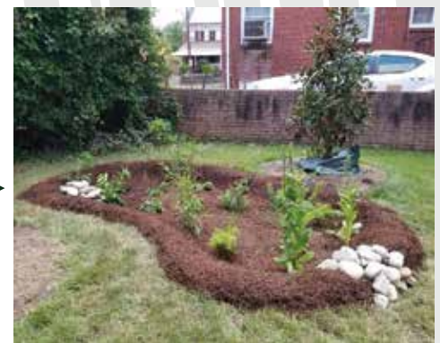
Downspout point of entry is protected to avoid channeling of water. Overflow area may also be protected if needed.
