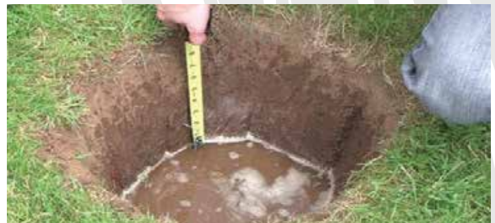
Perc test required to ensure adequate drainage. Water must drain within 36 hours.
