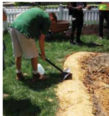
Compact level berm allows water to pool for up to 48 hours to slowly infiltrate water into ground.
